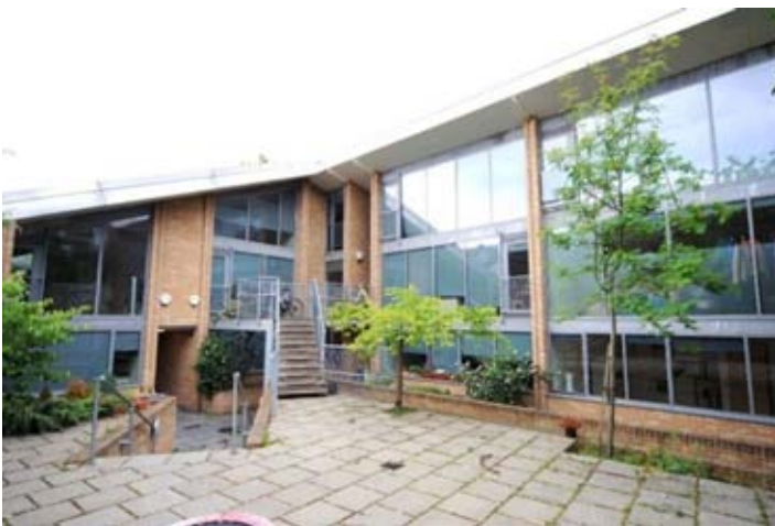
N19 Cornwallis Road 32878142 Litch- fields 2 Y N Balcony, New Build 285000
