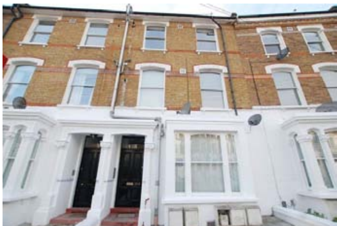
N4 St Thomas's Road 32079074 Next Move 2 N N 315000
