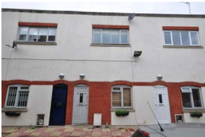
N16 Stoke Newington Road, Dalston 18022536 Douglas Allen 2 Y Y Freehold, house 295000
